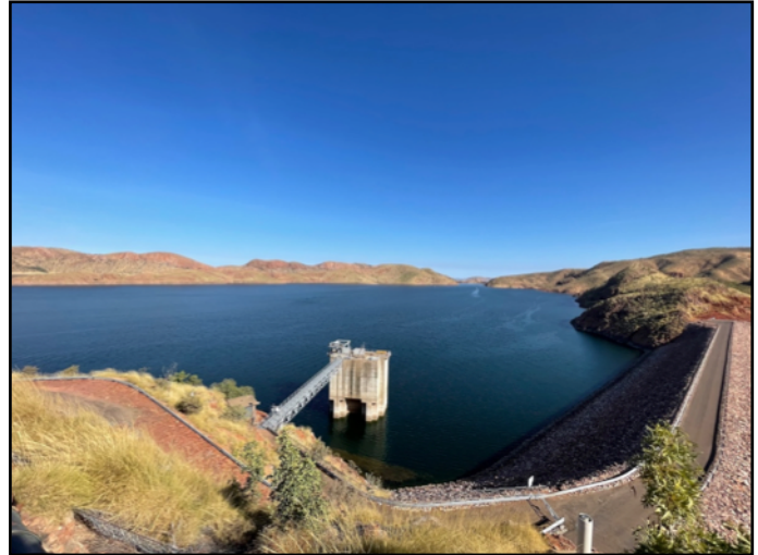
Ord River Dam, Kunanurra, NT
