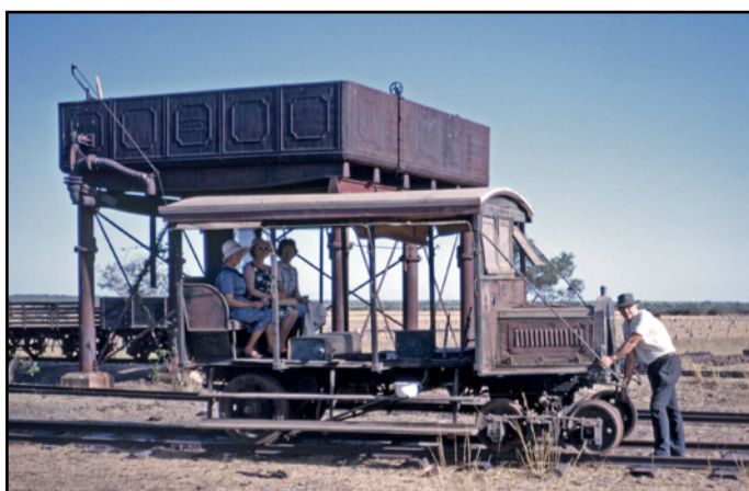
On 19 August 1964 the Officer-in-Charge of the Normanton-Croydon railway (Queensland) poses in front of RM14, a railcar that had been converted from a Panhard-Levassor car in 1918. It had just been rolled out of a shed where it had rested since its last ran in 1938. The occasion was a visit by a party of 20 from the Australian Railway Historical Society, Victorian Division
