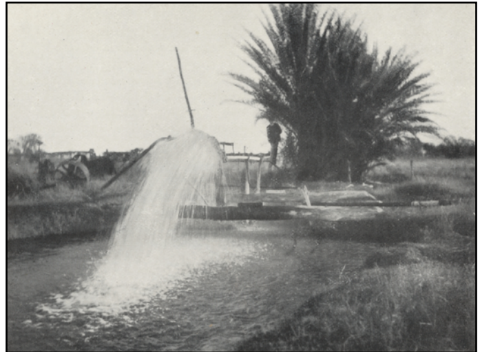
A bore in Northampton Downs. This bore has a daily flow of 100,000 gallons
